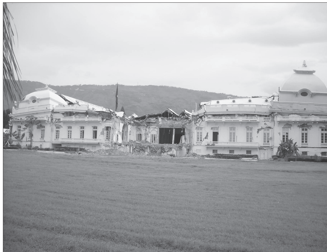
Damage caused by the Haitian earthquake of 2010 is still obvious throughout Port Au Prince, the nation's capital city. PHOTOS COURTESY OF HELPING TO HEAL HAITI
